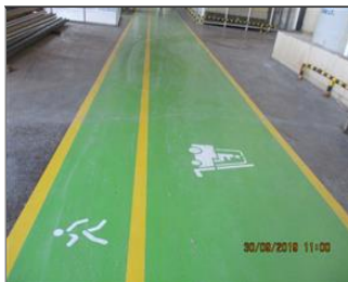
Photo of fire safety equipment Evacuation routes.JPG
