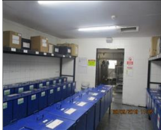
Photo of chemical storage room (if applicable) Chemical storage area (2).JPG
