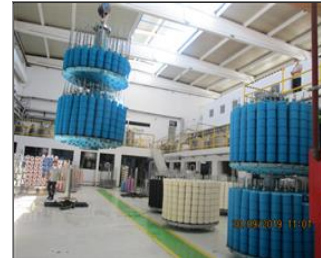
Photo of the inside of the main production hall Yarn dyeing area.JPG
